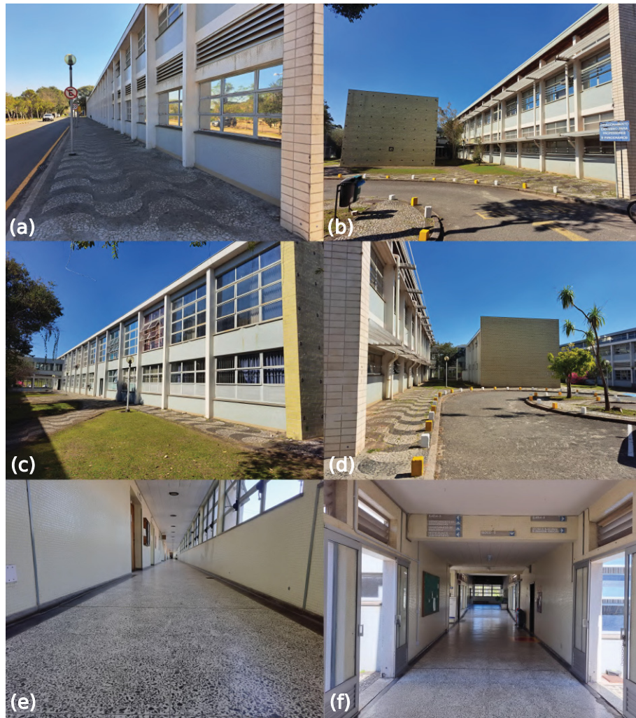
Figura 6.9: The environment used to build the database during the mobile robot's locomotion. Different surfaces and architectures were considered along the path, outdoor environment: (a) similar architecture, long distance for sensor measurement, and linear trajectory; (b) different architectures, parking, and irregular trajectory; (c) proximity between the walls on both sides and transition with the indoor environment; (d) different architectures, parking, and irregular trajectory; indoor environment, (e) narrow aisle for linear trajectory and measurement with left and right side sensors. Figure (f) shows the easy transition between indoor and outdoor environments through two side doors.
