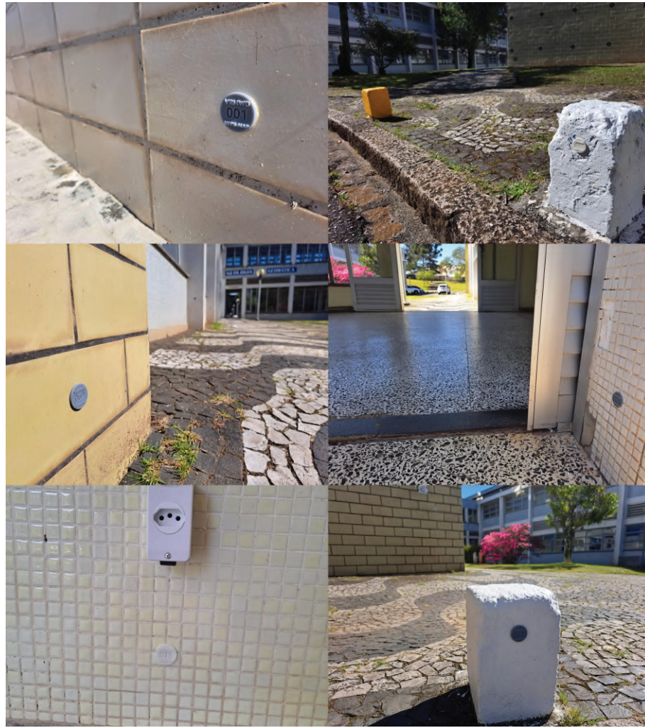
Figura 6.8: Tags fixed to the wall and pillars around the Geology building at the Federal University of Paraná - Polytechnic Center. The tags were positioned at an approximate height of 200 mm from the floor and tried to follow the architecture of the building to place the tags on each column or pillar, representing an approximate distance of 3 meters between the tags.
