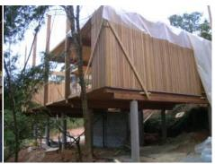
FIGURA 102 - PAINÉIS DE VEDAÇÃO (VILA TAGUAÍ). FONTE: ITA CONSTRUTORA (2010)
