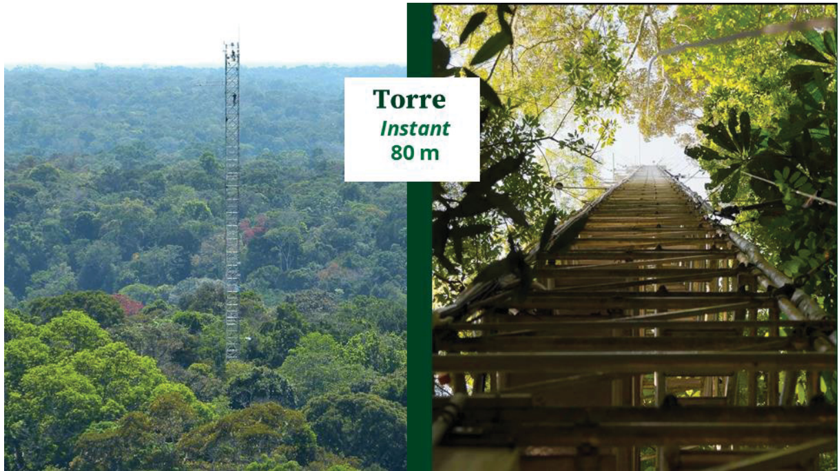
FIGURA 2 – TORRE INSTANT - WALK-UP TOWER
