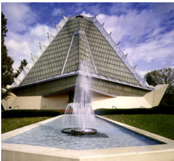
FIGURA 84– Sinagoga Beth Sholom de Frank Lloyd Wright (FONTE: VITRUVIUS, 2009)
