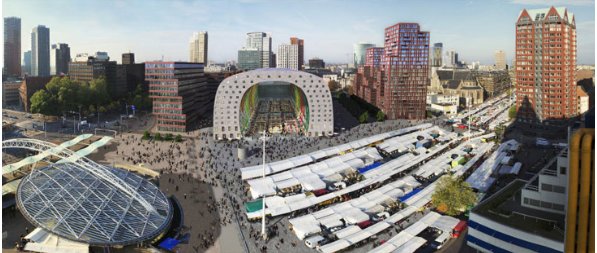
Figura 24 Rotterdam Market Hall
