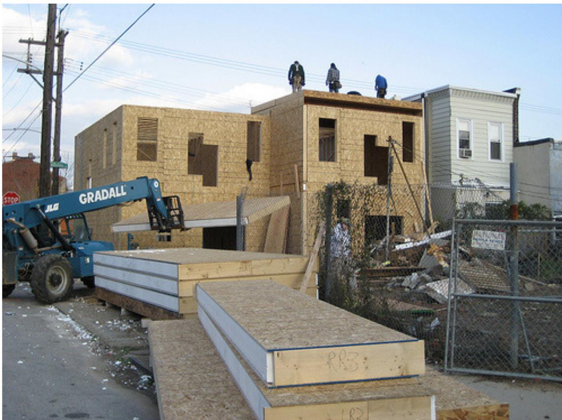
**Fig 3.27** – Cobertura isolante, sistema SIP - *Structurally Insulated Panel*.
