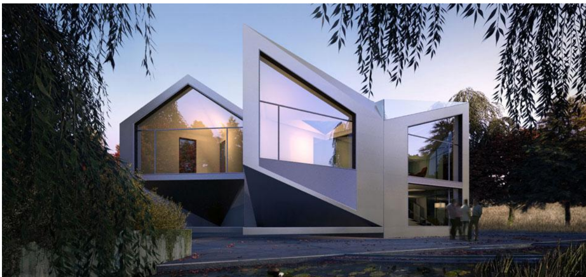
Figura 20: Vista exterior (THEDHAUS, 2013).
