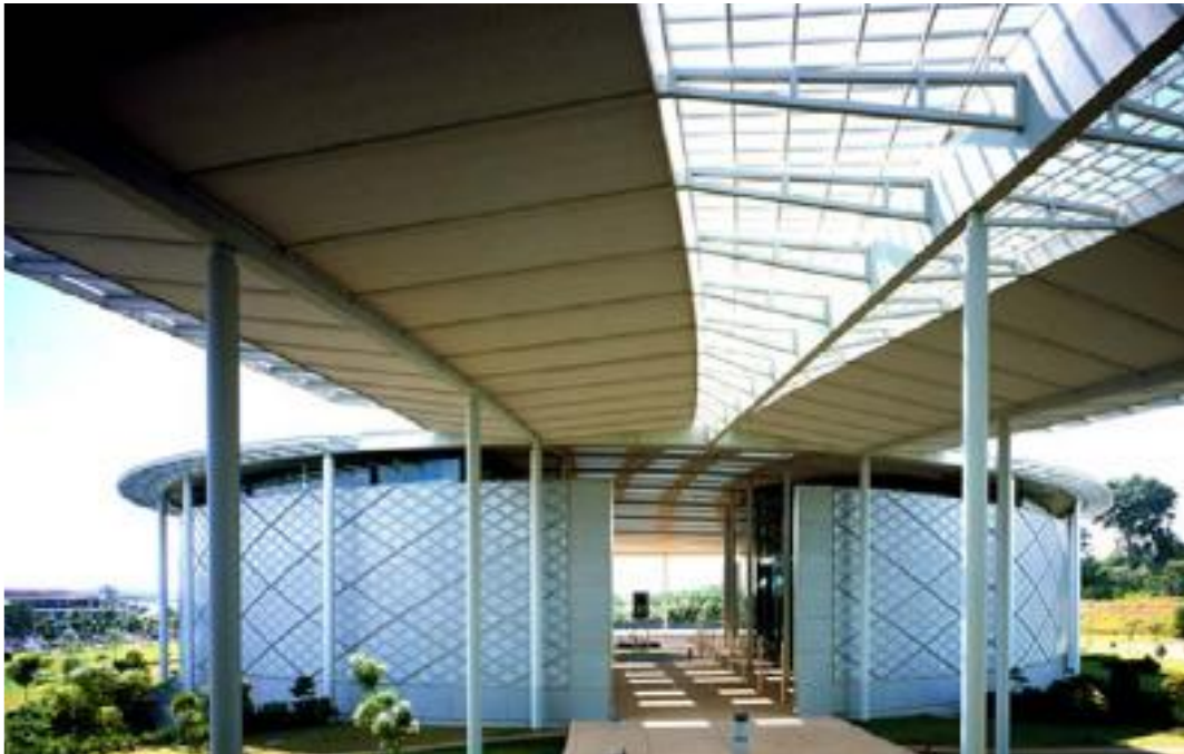
39 Vista do chancelor complex
