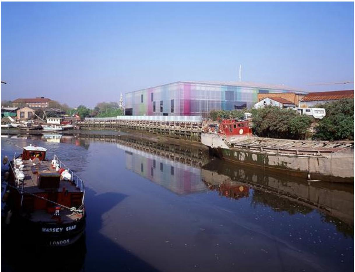
FIGURA 4.3 - LABAN AO FUNDO. OS PAINÉIS DE POLICARBONATO COLORIDOS DÃO LEVEZA E RITMO À FACHADA.
