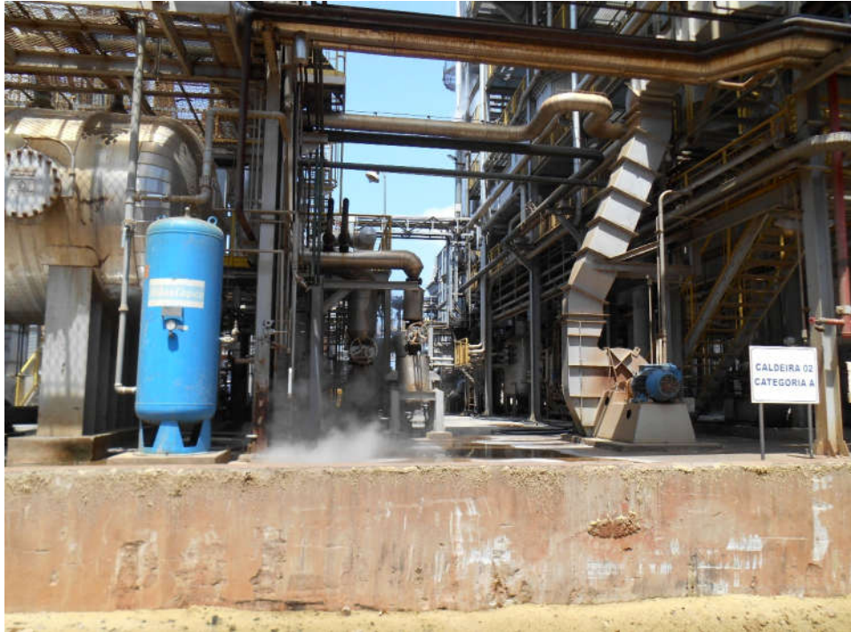
Foto: Douglas A. Aguiar. Usina Iacanga, out. 2014.
