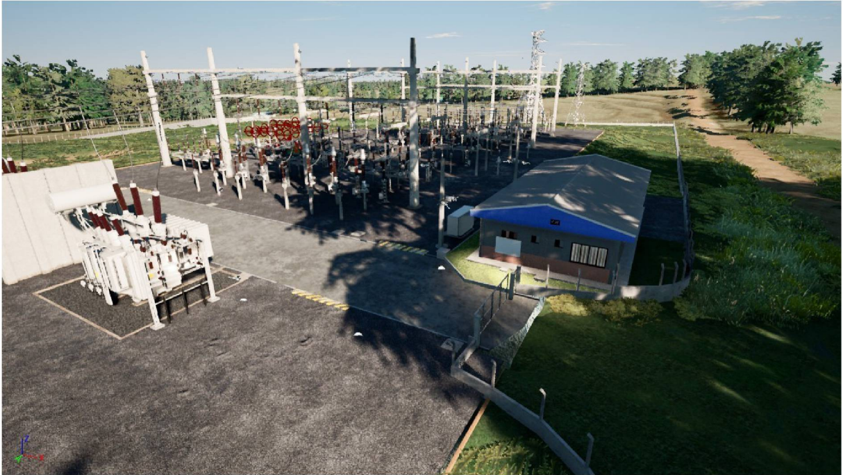
FIGURE 18 – An aerial view of the virtual environment, with the substation equipments modelled and placed as in the real environment. Source: OneReal research group.
