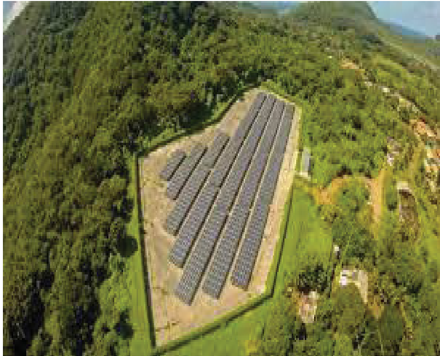
FIGURE 23 - NORONHA II SOLAR PLANT
