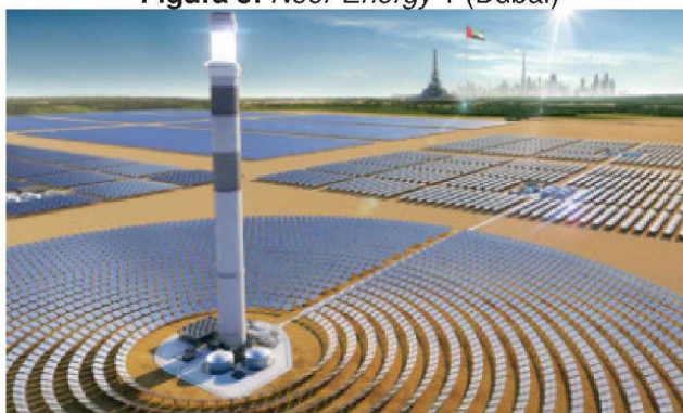
Figura 8: Noor Energy 1 (Dubai)
