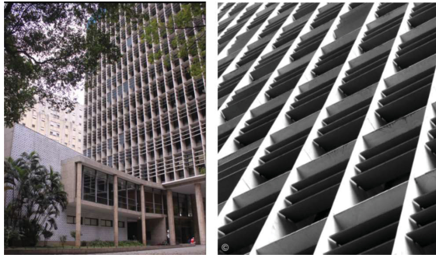
FIGURE 3 – BRISE SOLEIL EXAMPLE: MINISTRY OF EDUCATION AND HEALTH IN RIO DE JANEIRO, BY LE CORBUSIER AND OSCAR NIEMEYER, BRAZIL
