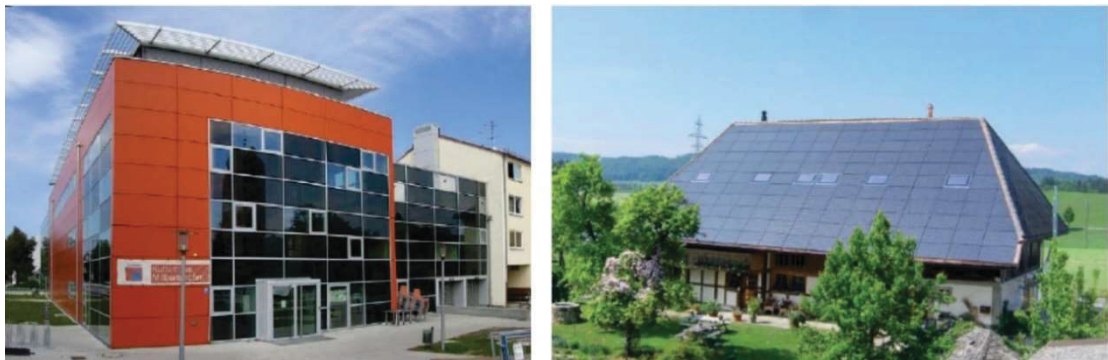
FIGURE 10 – BIPV APPLICATIONS: FAÇADE (LEFT); AND ROOF AS SHINGLES (RIGHT)
