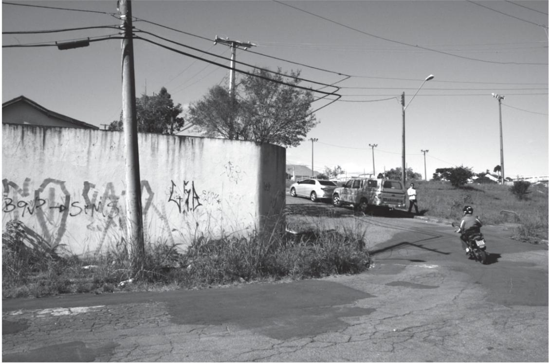
FIGURA 3 – ASFALTO COM DIVERSOS REPAROS
