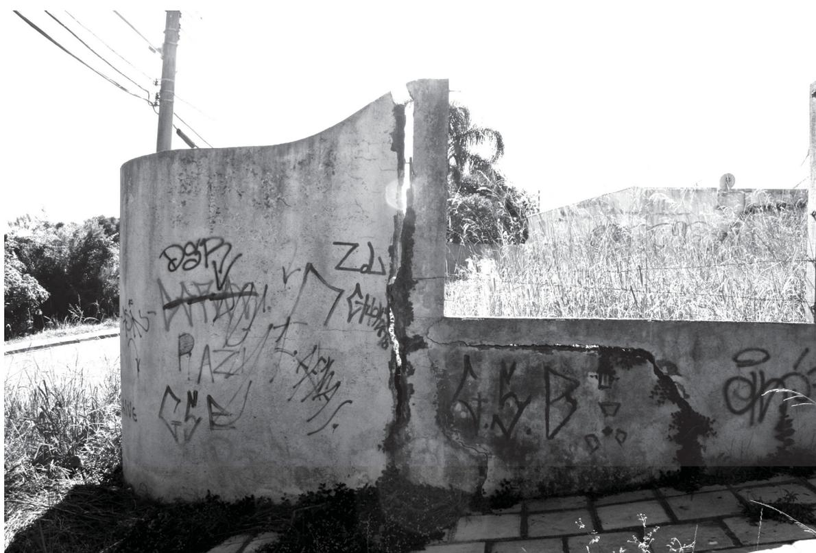
FIGURA 1 – FENDA NO MURO DE UMA RESIDÊNCIA
