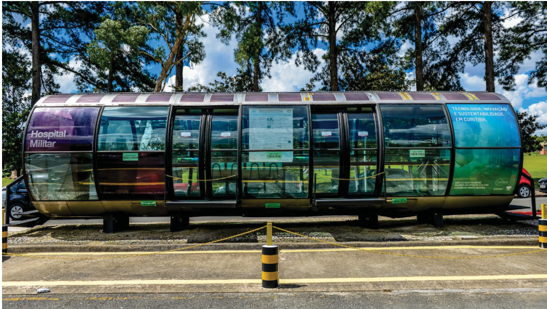
FIGURE 1.4: Tubelike station donated by URBS at Centro Politécnico/UFPR. OPV panels installed on the roof of the station
