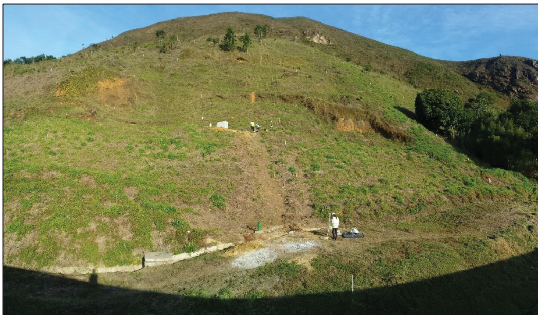
FIGURA 3.4 – TALUDE DO KM 552 PN
