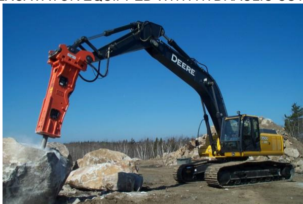
FIGURE 6 - EXCAVATOR EQUIPPED WITH HYDRAULIC CUTTER/HAMMER
