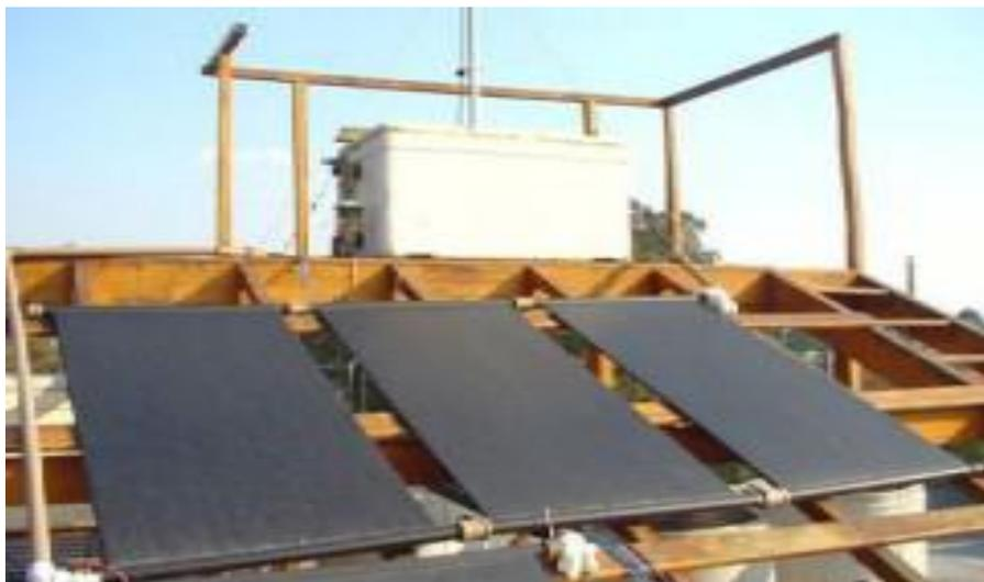
FIGURA 2.3: AQUECEDOR SOLAR DE BAIXO CUSTO (ASBC) DE WOELS E COLETOR SOLAR DE BAIXO CUSTO (CSBC).
