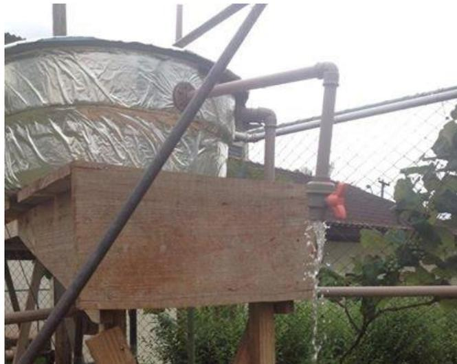
FIGURA 3.3: CAIXA D'ÁGUA ENVOLTA COM MANTA TÉRMICA.
