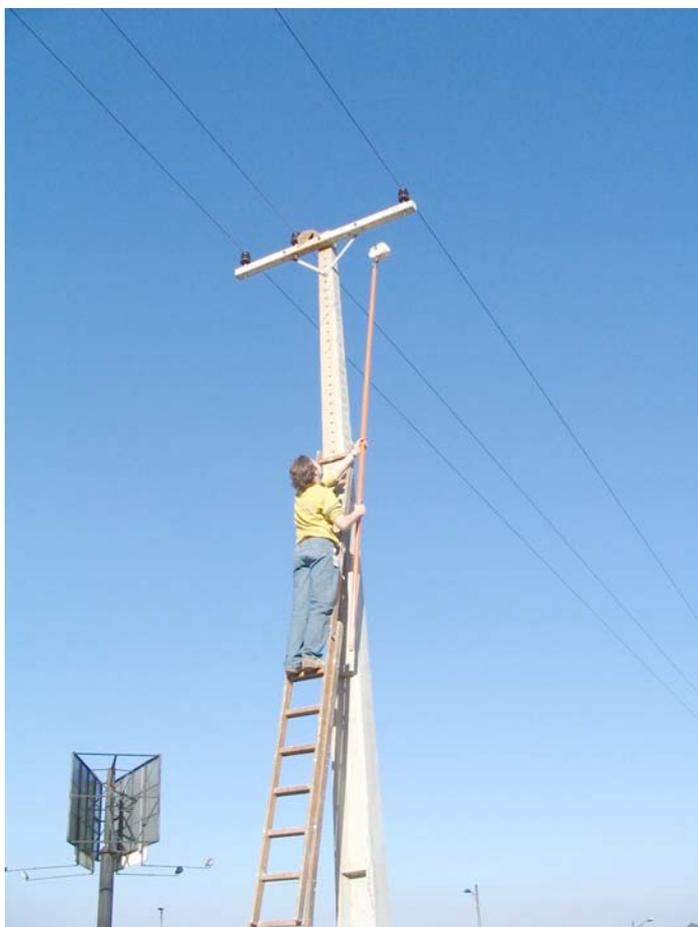
FIGURA 28 - FOTO DO SENSOR INSTALADO NA REDE EXPERIMENTAL
