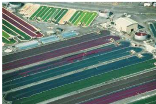
Figure 5. 90 acres commercial microalgae production facility, Kona, Hawaii. Note: green ponds culturing Spirulina and red ponds with Haematococcus pluvialis .
