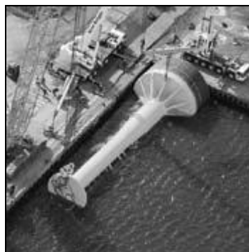
Figure 6-17: Bucket foundation at transport (BLADT, 2010)
