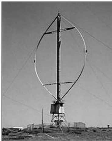
Figure 5-5: Darrieus-rotor (left) and H-Darrieus-rotor (right) (WIKIPEDIA, 2009)
