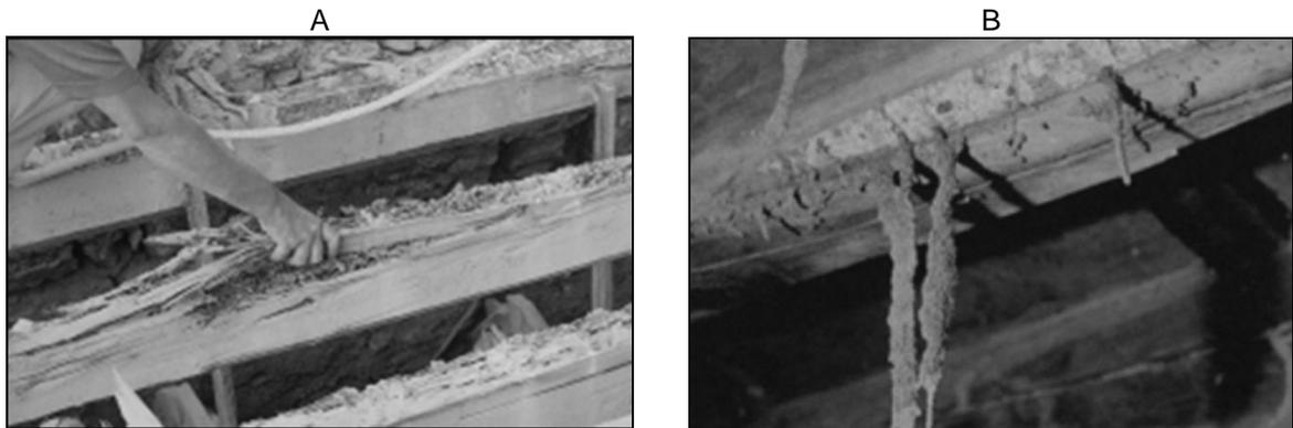
FIGURA 30 – CUPINS-DE-MADEIRA-SECA EM COBERTURA (A)
