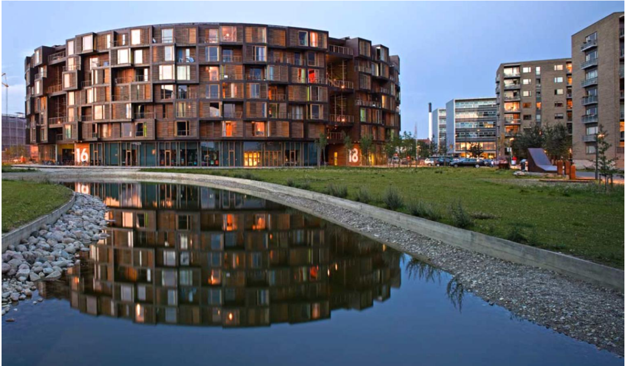
Figura 3.11 Tietgen Hall of Residence FONTE: NYT, 2008.
