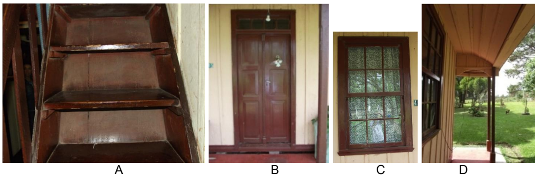
FIGURA 29 – ESCADA (A), PORTA (B), JANELA (C), FORRO (D).
